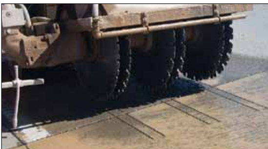
Cutting the slots (sawing).
