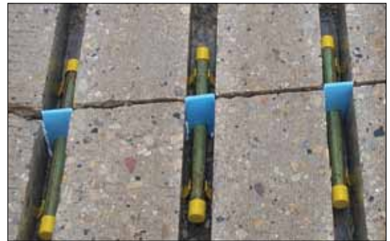
Placing the dowel bars, caps, chairs and joint filler.
