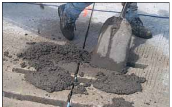
Backfilling the slots with DB Retrofit Mortar.
