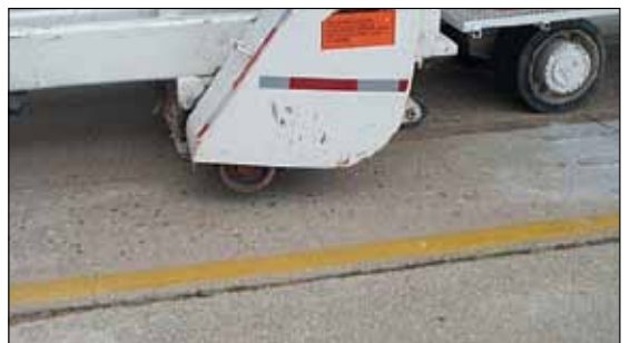
Diamond grinding of pavement lane.
