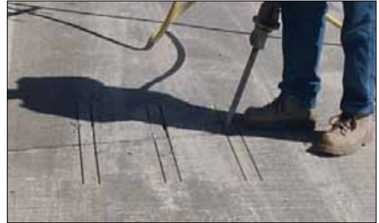
Preparing the slots.
